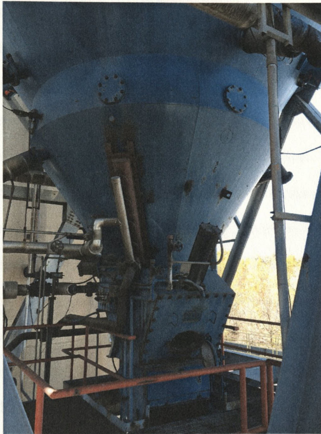
Figure 9 - Existing Dewatering Bin Unloading Cone and Equipment
