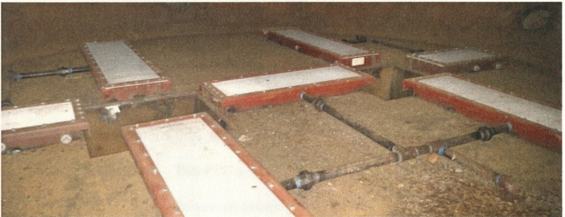
Figure 17 - Installed Fluidizing Stones Inside of Silo on New Flat Bottom
