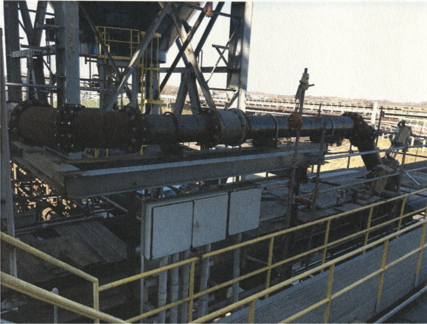
Figure 13 - Fly Ash Transfer Tie-In Piping
