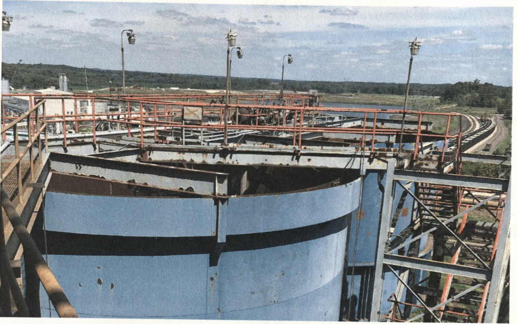
Figure 6 - Top of Existing Dewatering Bins Prior to Demolition
