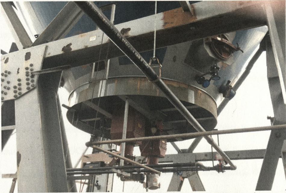
Figure 12 - New Tank Bottom Installation During Construction
