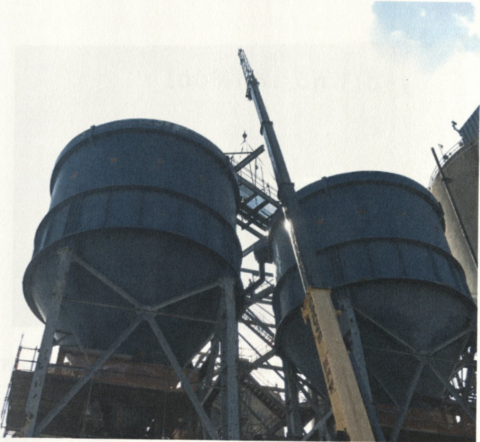
Figure 7 - Existing Dewatering Bins During Demolition of Platforms
