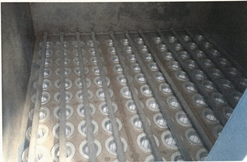
Figure 14 - Interior Photo of the New Baghouse Collection Device
